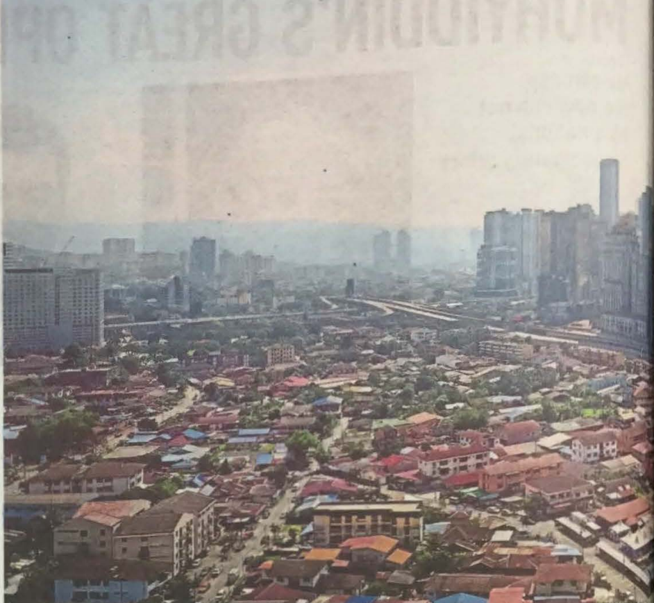
Kampung Baru in Kuala Lumpur. The government is urged to update landowners on the type of groundwork that will be done on the massive redevelopment project involving 80ha in the enclave. FILE PIX
