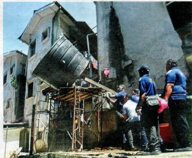
DBKL officers demolishing the water tank in Jalan Beremi, Kuala Lumpur.
