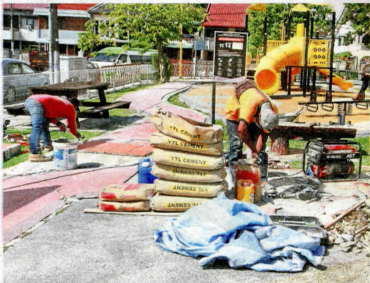
Workers laying out the new pavement next to the playground in Taman Batu.
