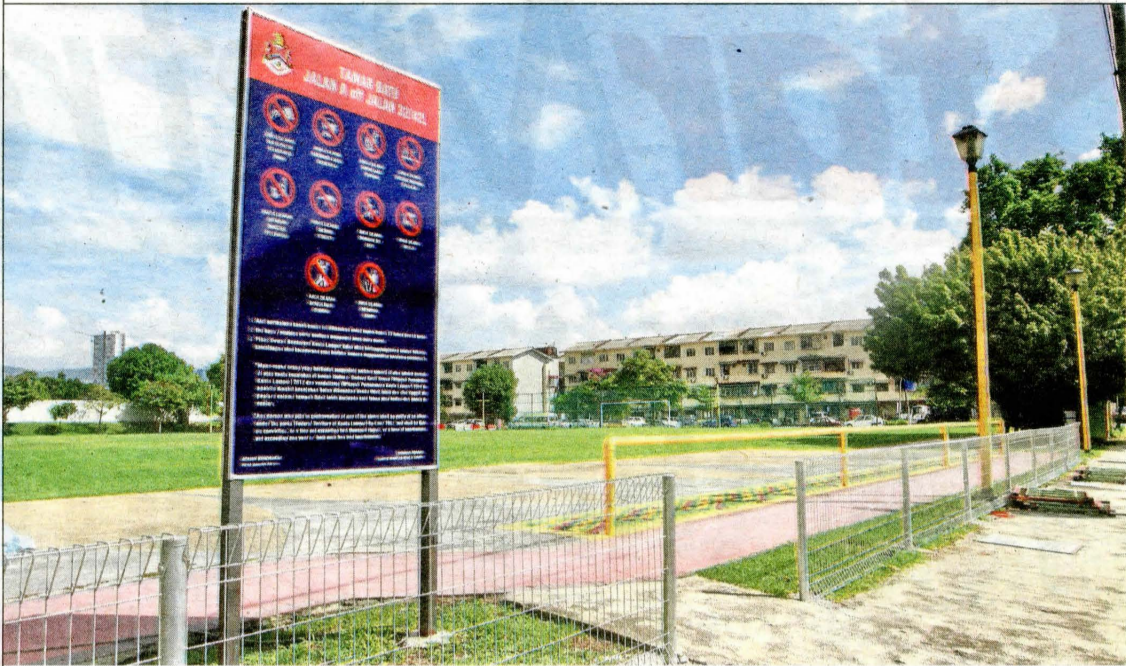
Upgrading work is ongoing at the football field at Jalan A off Jalan 32/42L in Taman Batu, Kepong. — Photos: LOW LAY PHON/The Star
