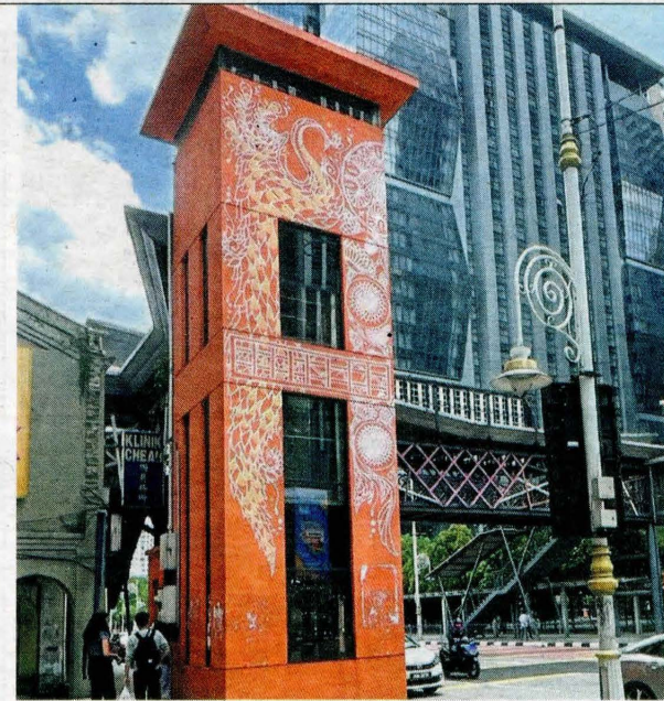
The lift shafts along Jalan Tun Sambanthan take up a big portion of the walkway. Some stakeholders want the lift shafts removed but the foot bridge to remain. — Filepic
