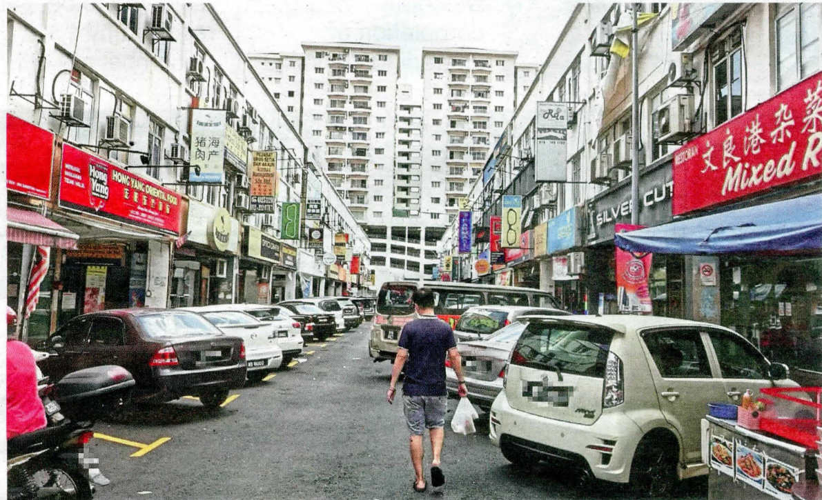
Roads have been retarred and the faded road markings repainted at Prima Setapak, Kuala Lumpur.
