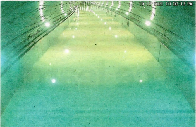
Inside the SMART Tunnel during Mode 4.
