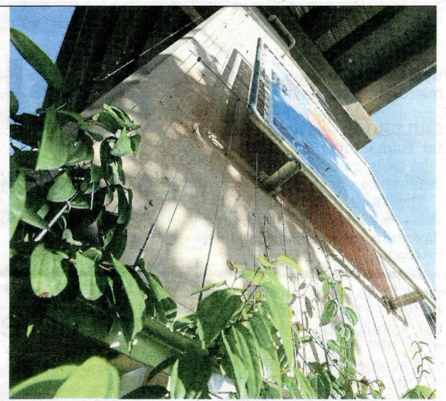
Steel frames installed on Duke 2 pillars to encourage the growth of creepers.
