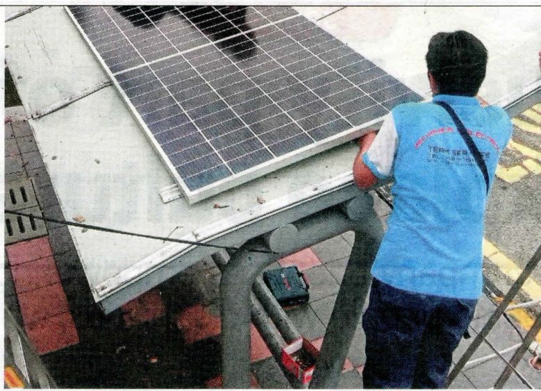
A DBKL contractor installing solar panels on a bus stop's roof in Wangsa Maju.
