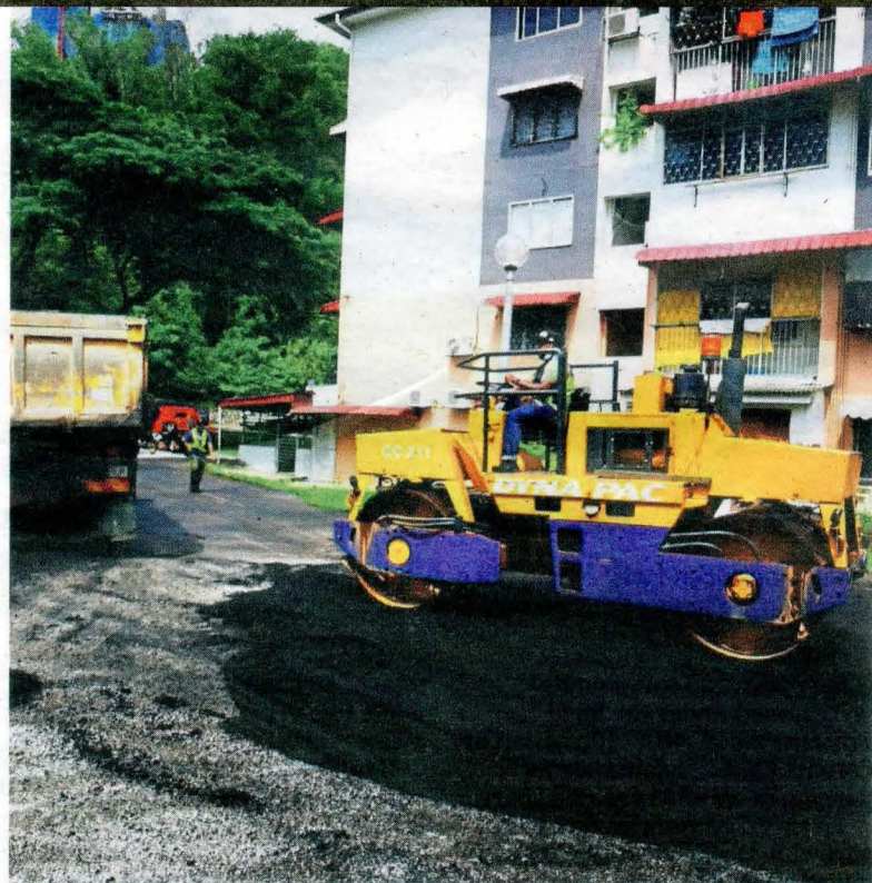
DBKL resurfacing roads under its jurisdiction at the Wangsa Maju flats.
