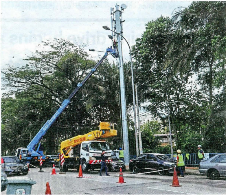
A telecommunication tower being installed in Taman Desa, Kuala Lumpur.
