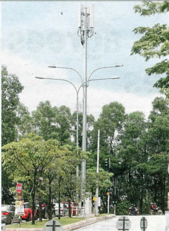
A hybrid telecom and lamp post along Jalan Senang Ria, Kuala Lumpur. – FAIHAN GHANI/The Star
