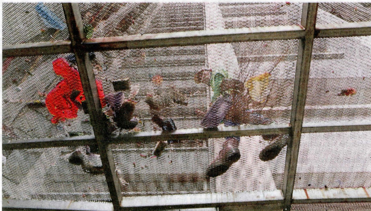
DBKL installed netting to prevent dangerous objects from falling below at PPR Seri Pantai, Kuala Lumpur.
