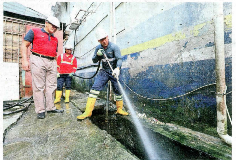
Mohd Zain (left) observing an Alam Flora worker having to manoeuvre his way around to clean the drains in Pudu.
