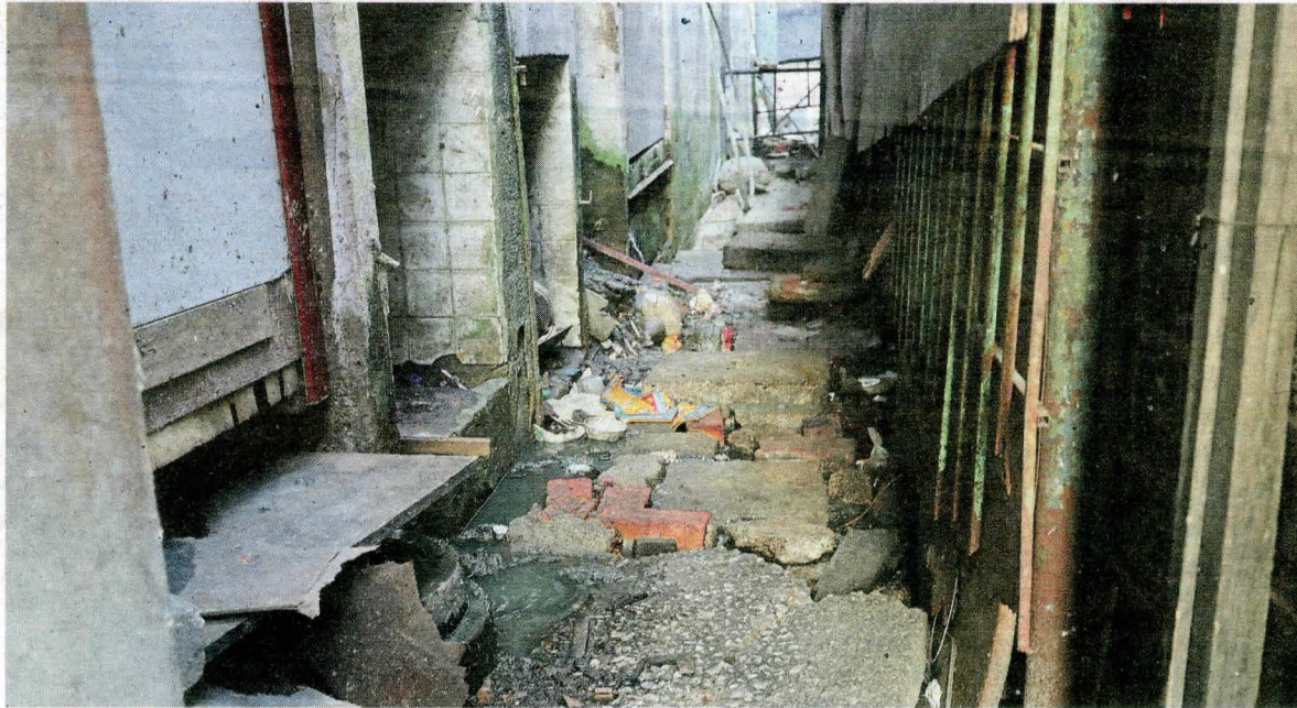
This side lane in Bukit Bintang, previously wide, has been reduced to a narrow lane due to many illegal extensions.
