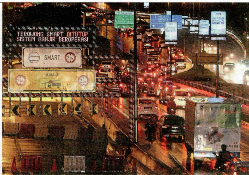
The SMART Tunnel closed to traffic following a downpour to divert stormwater. – Filepic
