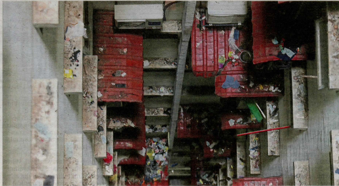
Rubbish and other items thrown out of windows can be seen on awnings and ledges of PPR Sri Aman's airwell in Kepong. — YAP CHEE HONG/The Star
