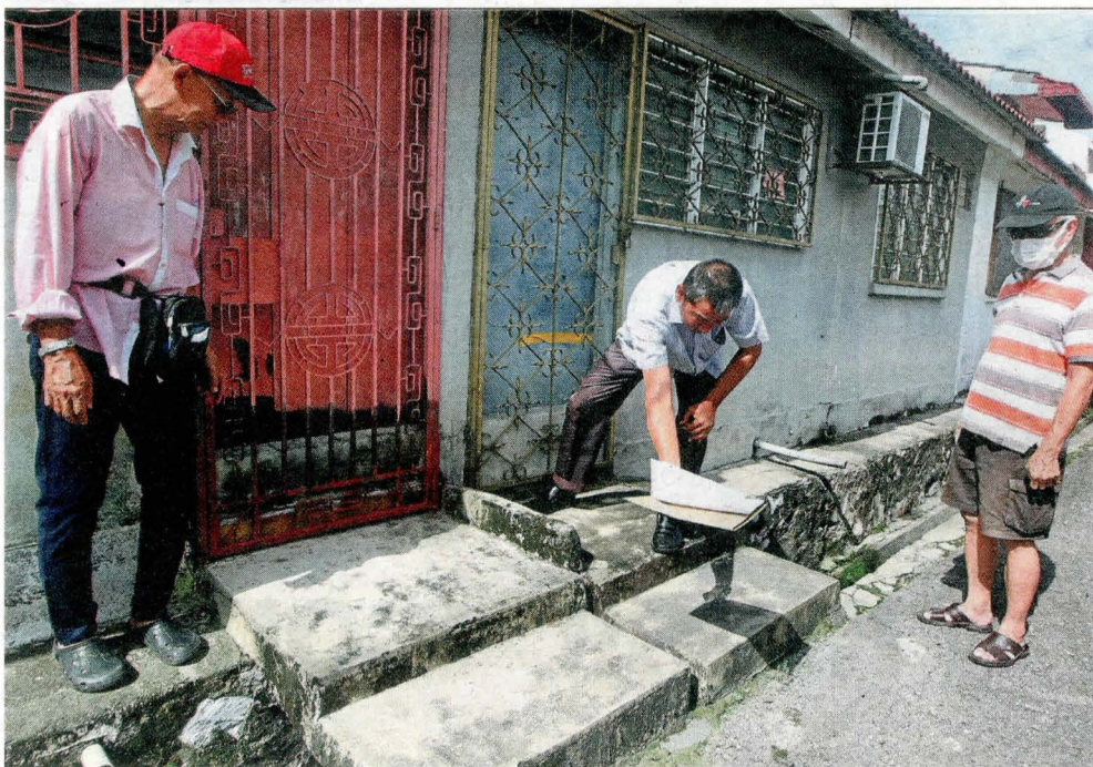
Yee (centre) showing how high the floodwater rises during heavy rain. — KAMARUL ARIFFIN/The Star
