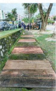
Boo provided the photo of broken and missing drain slabs in Jalan 4/91 in Taman Shamelin Perkasa to DBKL and when contacted by StarMetro, DBKL showed (right) that it has installed wooden slabs over the monsoon drains as a temporary measure.
