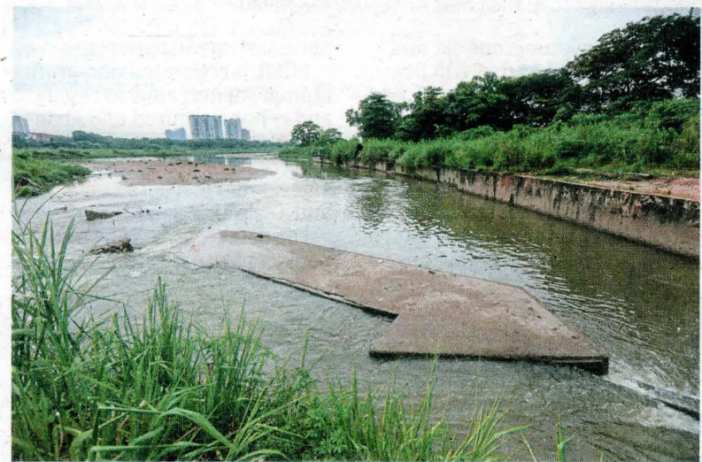
The Bohol flood retention pond in Seputeh is one of 15 in Kuala Lumpur. — Filepic
