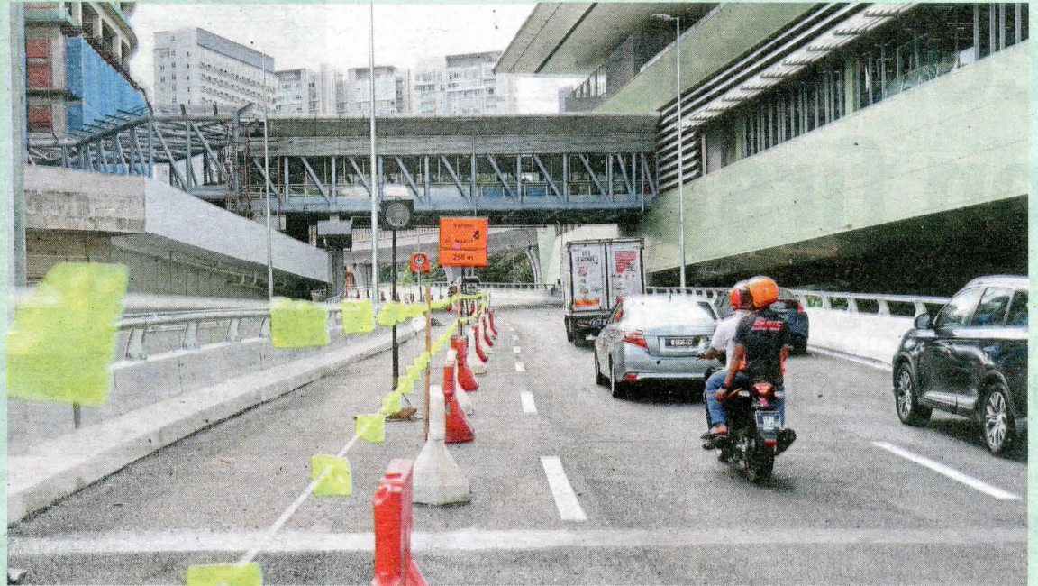
The flyover from Jalan Maarof to Jalan Semantan in Bangsar can now be used. — ART CHEN/The Star
