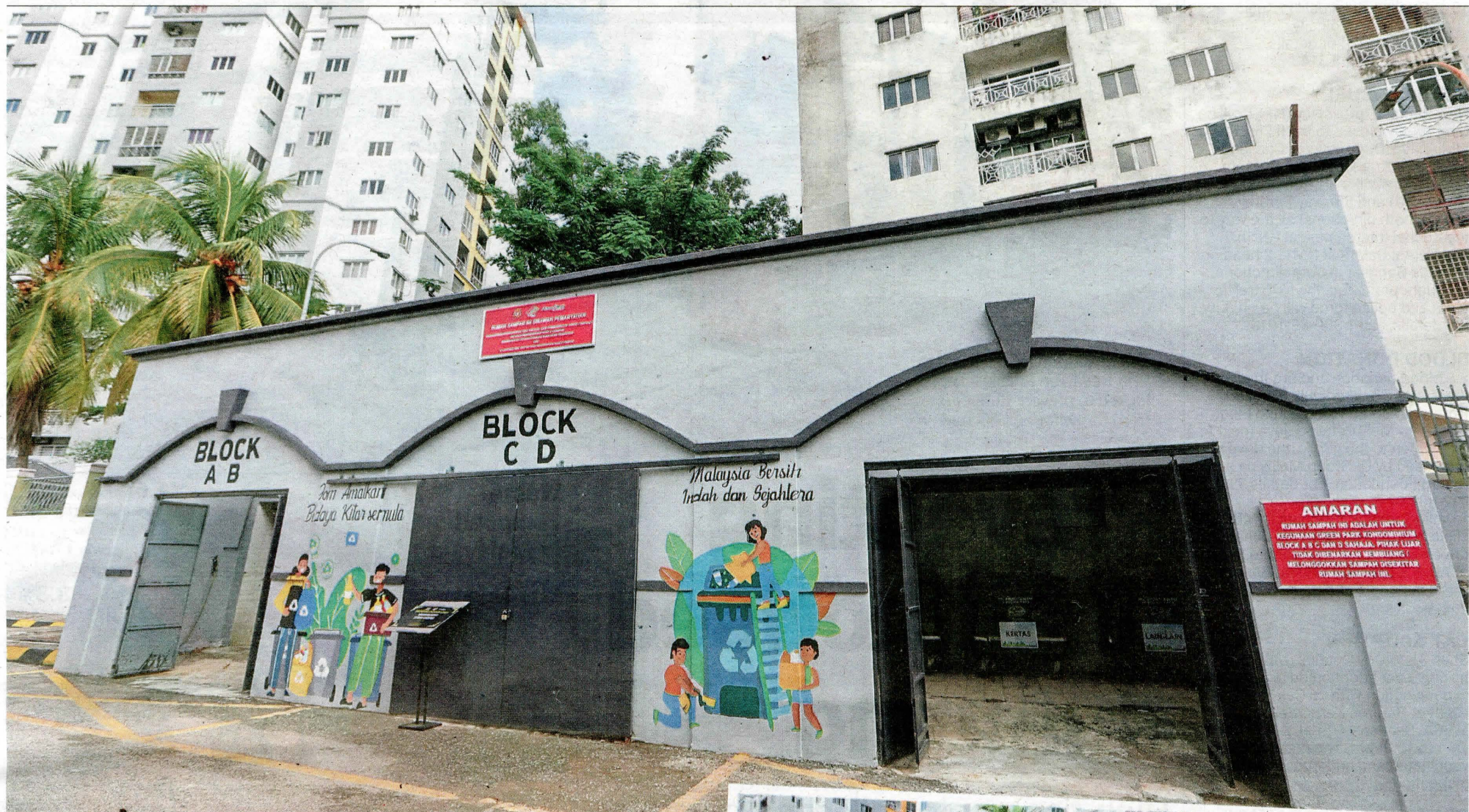
A refuse room that has been cleaned up and given a new coat of paint at Green Park Condo in Jalan Awan Pintal of Taman Yari, Kuala Lumpur. (Right) Its condition before refurbishment. — Photos: YAP CHEE HONG/The Star
