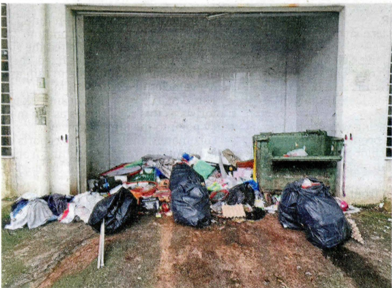
The refuse room at Wisma OUG in Jalan Cempaka before (left) and after its transformation.
