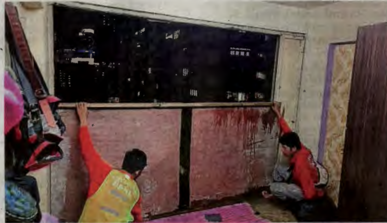
DBKL contractors temporarily fixing a wall that was ripped out by strong winds at Loke Yew flats.
