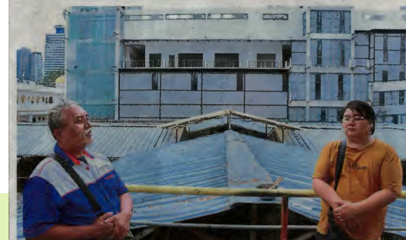
Yuesnaedy (left) and Chew with the 95%-completed phase two complex behind them.
