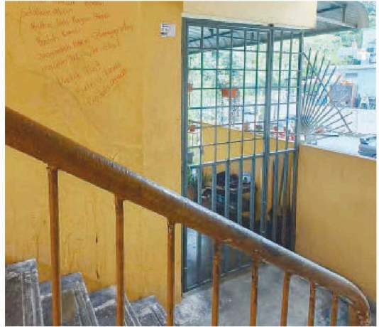
This safety grille, which impedes access to the common corridor and blocks access to safety in the event of a fire, has riled some residents, who left an angry message on the wall next to it.
