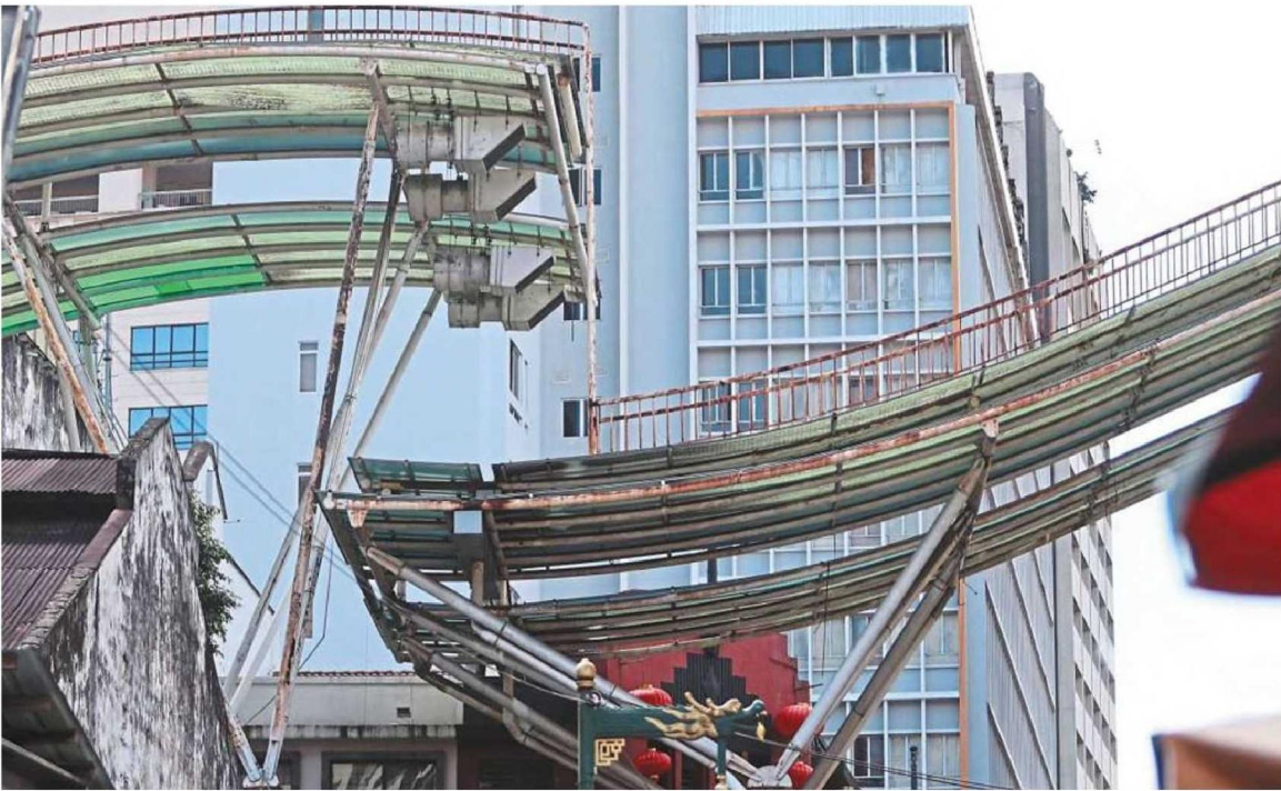
Upgrading works at Chinatown area including the roof are expected to start after Chinese New Year.
