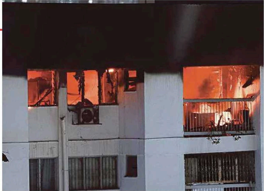
Fire engulfing units on the 17th floor of Block 70 at the Sri Sabah flats in Cheras, Kuala Lumpur, on Sunday night. BERNAMA PIC
