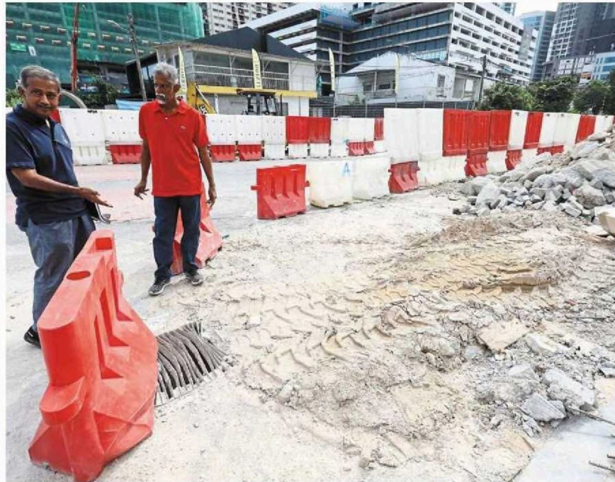
(Above) A loosely covered hole among dangers faced by pedestrians at the construction site.
