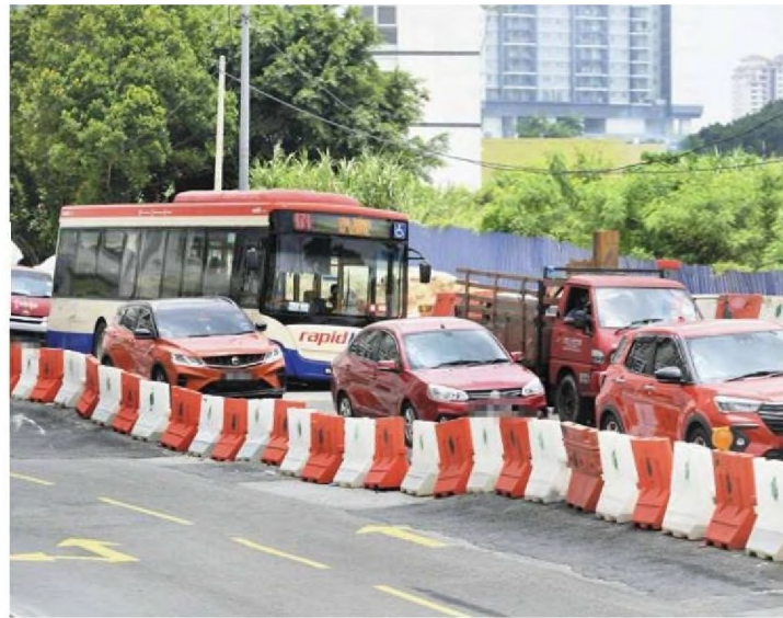
The uneven surface of Jalan Sentul Pasar. — ONG SOON HIN/The Star
