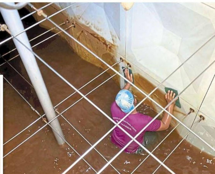
(Above) Cleaning work being carried out on a fibreglass-reinforced plastic tank. (Inset) A still from the viral video of sludge found at the bottom of a water tank.
