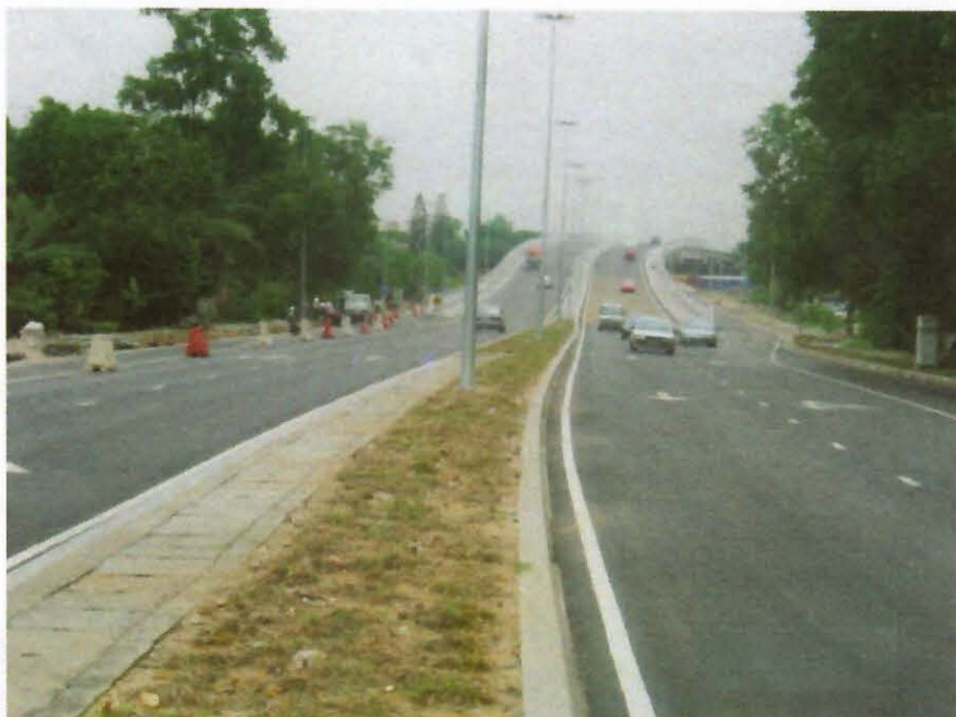
The new flyover linking Taman Kepong Baru with Taman Bukit Maluri is completed and was officially opened by Datuk Mohamad Shaid bin Mohd. Taufek, Mayor of Kuala Lumpur and Y.B. Tan Kee Kwong on 13 February 2004. Photo KL City News
