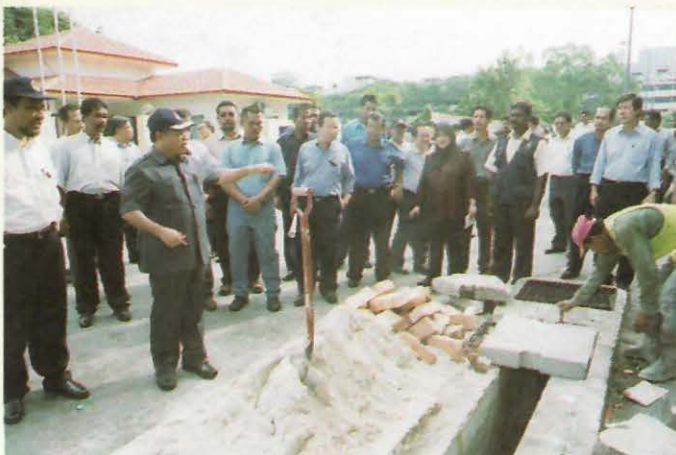
Covering open-drains with concrete slabs. - Photo KL City News
