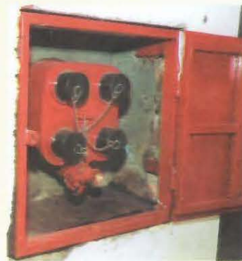
Wet riser fire hose outlet without fire hose
