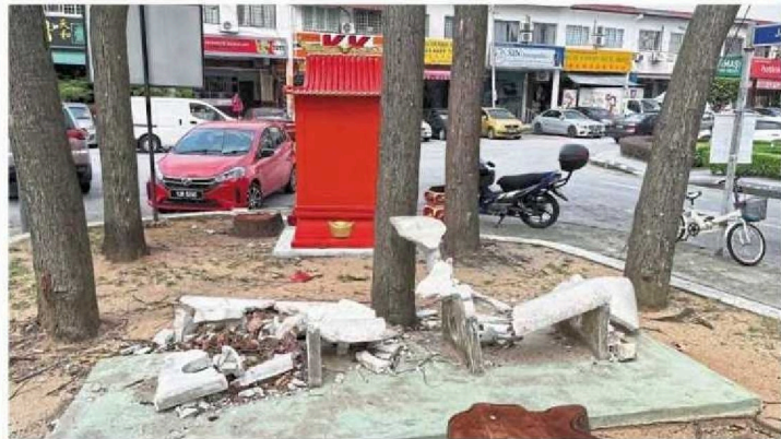
Damaged concrete benches in the Taman Baru Jinjang park.
