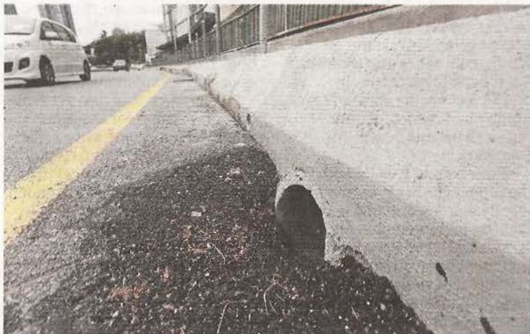
Scupper drains along Jalan Maarof, which are crucial for flood mitigation, have been unblocked.
