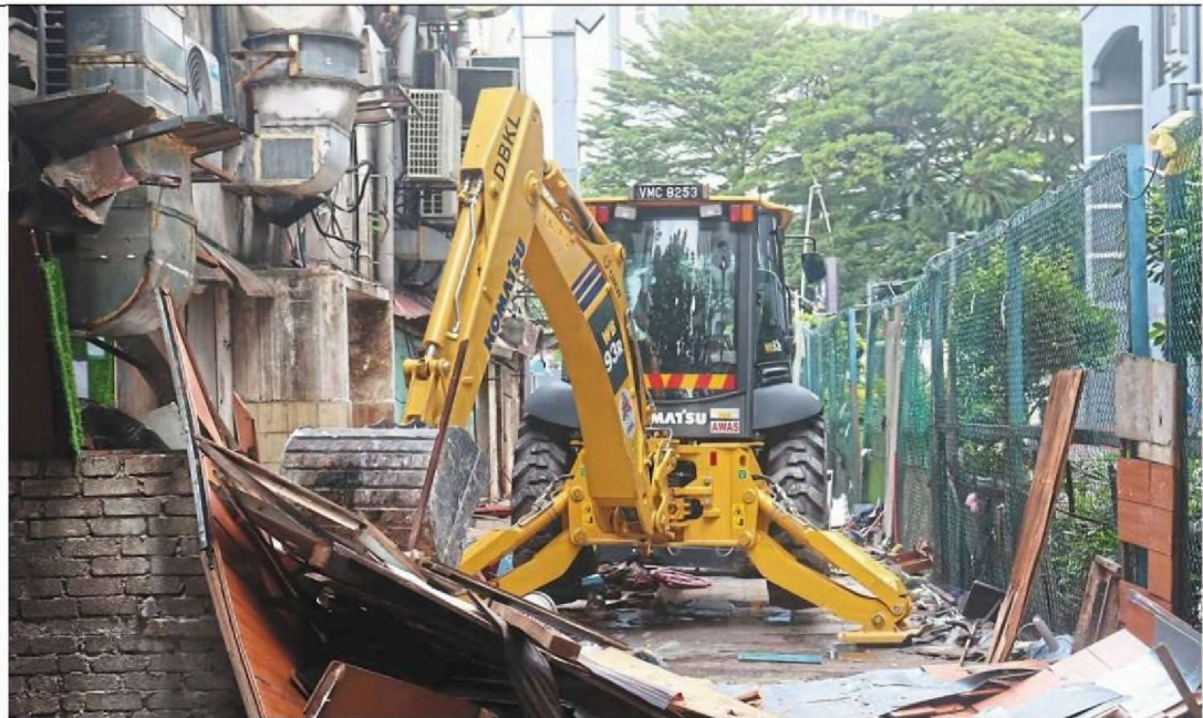
An excavator tearing down an illegal structure in the lane located behind Jalan Sultan, Kuala Lumpur.
