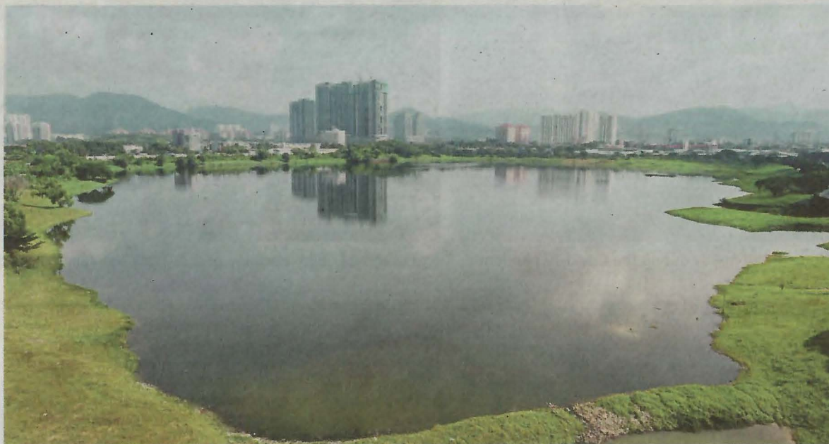
Retention ponds, such as the Batu pond in Kuala Lumpur, are vital assets to prevent flooding in the surrounding areas. — Filepic
