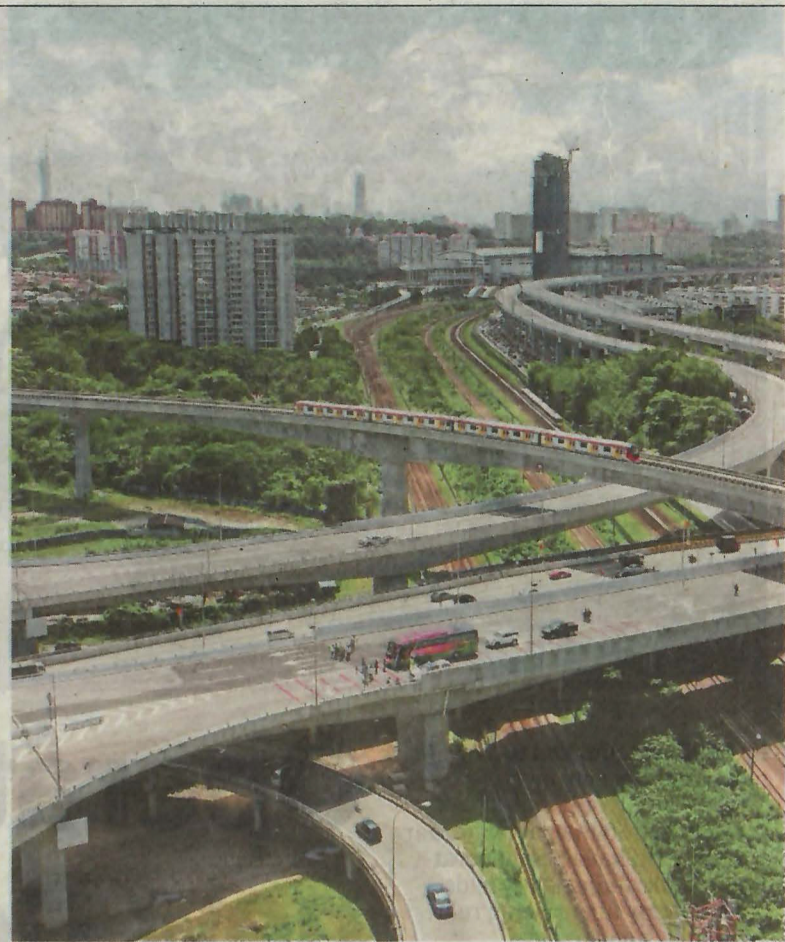
There is plenty of space beneath the recently opened Sri Petaling Interchange in the Sungai Besi-Ulu Kelang Elevated Expressway (Suke).
