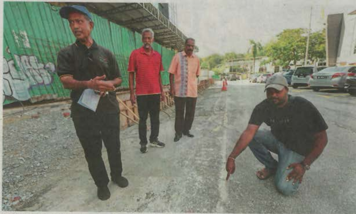
Ali (left) and Raju (second from right) with residents showing the markings of how far the project site had initially extended onto the street. — Photos: YAP CHEE HONG/The Star
