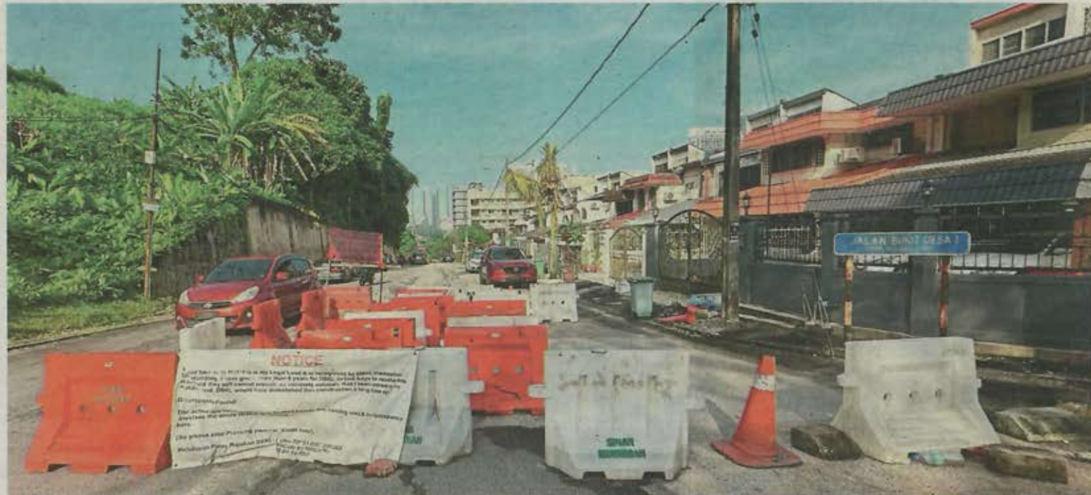
Barriers placed by Lim in front of his house in Jalan Bukit Desa 1. — MUHAMAD SHAHRIL ROSLI/The Star
