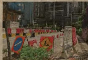
The site of the proposed pedestrian bridge in Jalan Rozario, Brickfields. — AFP/UMM
