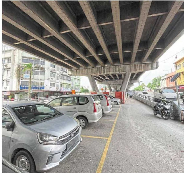
The mechanical parking bay project under the Jalan Yew-Jalan Sungai Besi flyover is awaiting DBKL’s approval. — LOW BOON TAT/The Star
