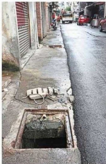
This drain behind Jalan Alor is on the verge of collapsing. (Right) Another lane in the Bukit Bintang area where several drains are without covers.
