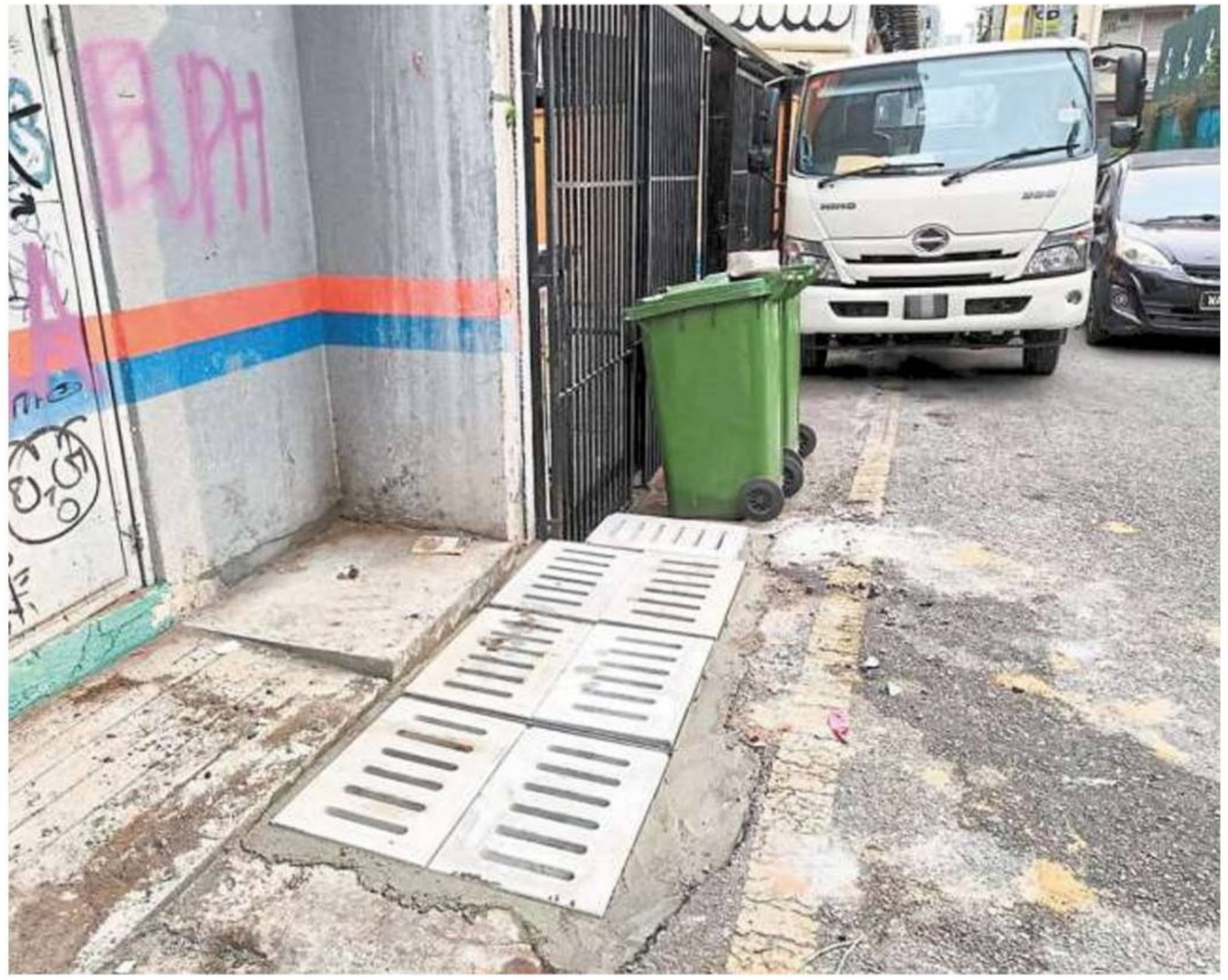
Drain covers before and after they were repaired in the back lanes of Jalan Alor in Bukit Bintang, Kuala Lumpur.
