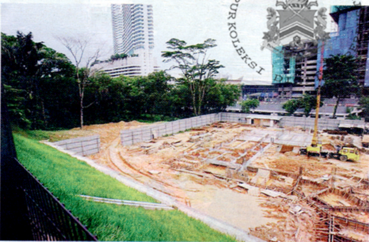
The designated land: The development taking shape on Federal Hill.
