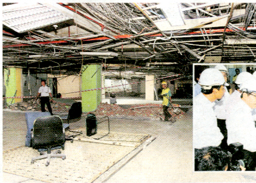
Workers to convert the mezzanine floor into the new waiting area. (Inset) Datuk Raja Nong Chik Raja Zainal Abidin (second from right) during a briefing on the Puduraya bus station. — Pictures by P.C. Lim
