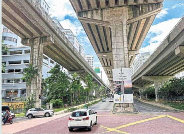
DBKL says it will upgrade and widen the roads linking Jalan Segambut Dalam and Jalan Kiara 4. — SHAARI CHEMAT/The Star
