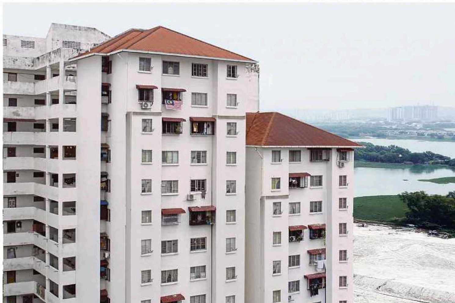
A graphically modified picture of a People's Housing Project in Kuala Lumpur. A resident of one project in the city says some residents own two cars, but refuse to pay the RM42 monthly maintenance fee. FILE PIC
