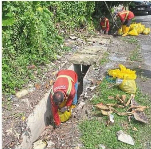
Alam Flora workers clearing out a drain along Jalan Jinjang Setia 6.
