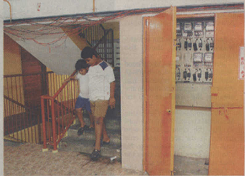
Danger: Wires hanging from the ceiling and an electric circuit box left open is upsetting residents.
