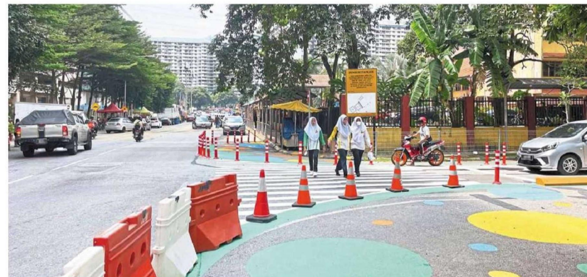
Before the full implementation of the new road design at SK Danau Kota 2, pop-up infrastructure such as lane separation cones are used to gauge its effectiveness.
