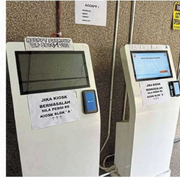
Several parking payment machines at the carpark are non-functional.
