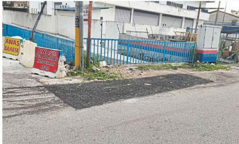
The sinkholes in Jalan Jinjang Aman 5 have been repaired.
