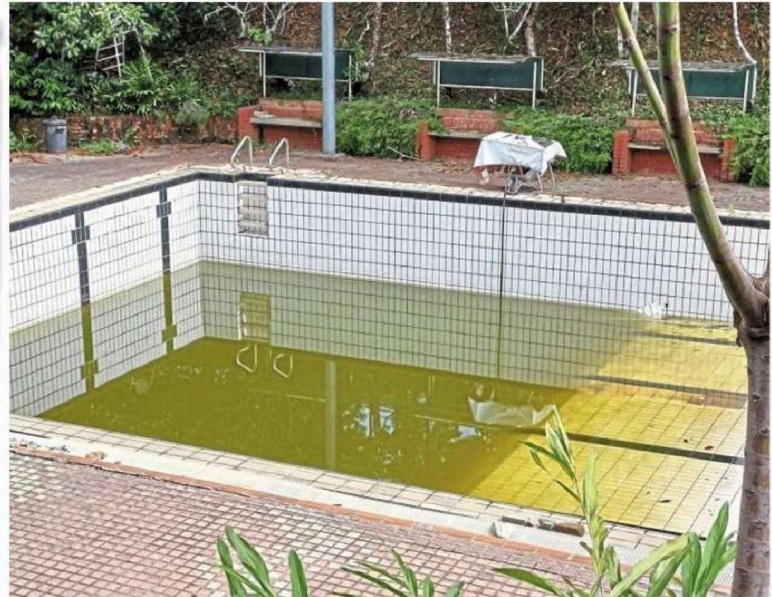
Murky water fills the once-busy 25m swimming pool at Bangsar Sports Complex in Jalan Terasek, Bangsar Baru. — Filepic
